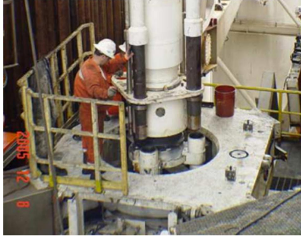
Figure 6 – Two riser joints are being connected in the spider [17].
