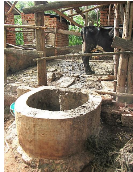
Figure 3: A part of the digester: the mixing tank. The cow shed can be seen in the background. (Source: Heidi Hustad Gleditsch)
