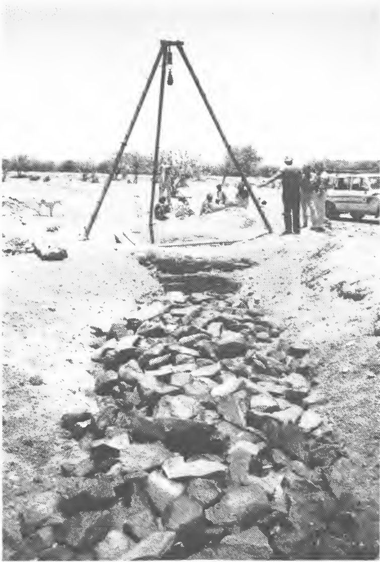
LEFT: Well Rehabilitation with infiltration ditches
