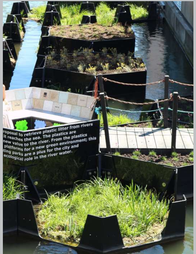
Fig. 4.35: Recycled Island Foundation
