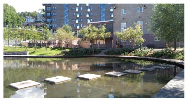
Figure 2.2(B) – Kværnerdammen is located on the Alna water course, at a former industrial site The pond basin is concrete, without emergent vegetation. It is vacuumed to remove algal growth. (Photo: July 2017)
