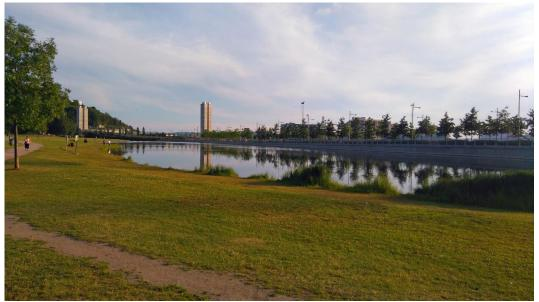
**Figure 2.3** In this photo of Vannspeilet (site B01), in Middelalderen park, a "hard edge" of concrete can be seen on the right side of the pond, below the pedestrian/cycle lane. The sloping lawn down to the water is a "soft edge".
