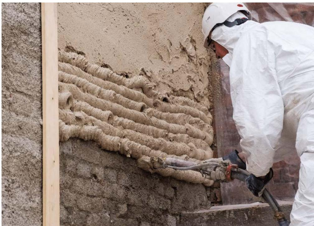
Figure 23- A worker applying Fixit222 with a spray gun ((Source: Boligbygg).
