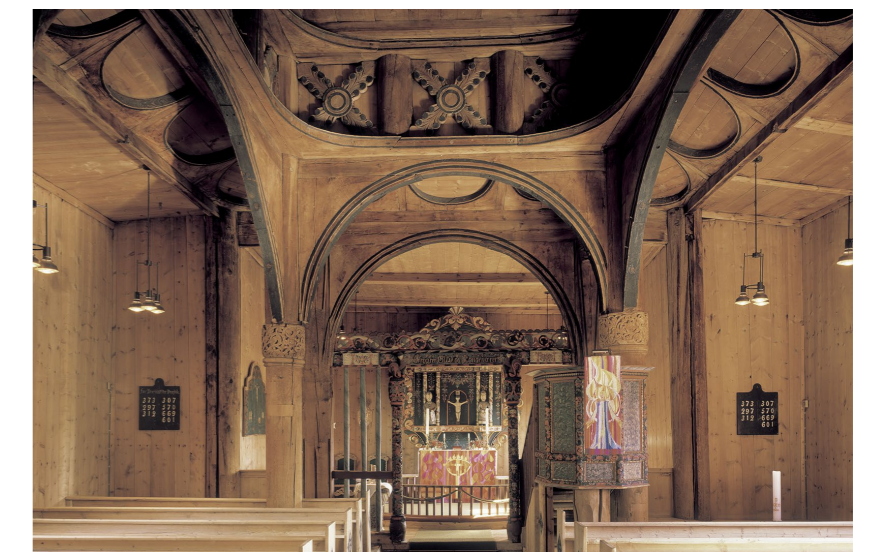
Fig 87. Anker, L. (2005). The technical construction details of an old stave church represents documentation or knowledge values (in its technical, and architectural historical value), the smell, color, perspective, material, and atmosphere constitute some of the experiential values of these highly
