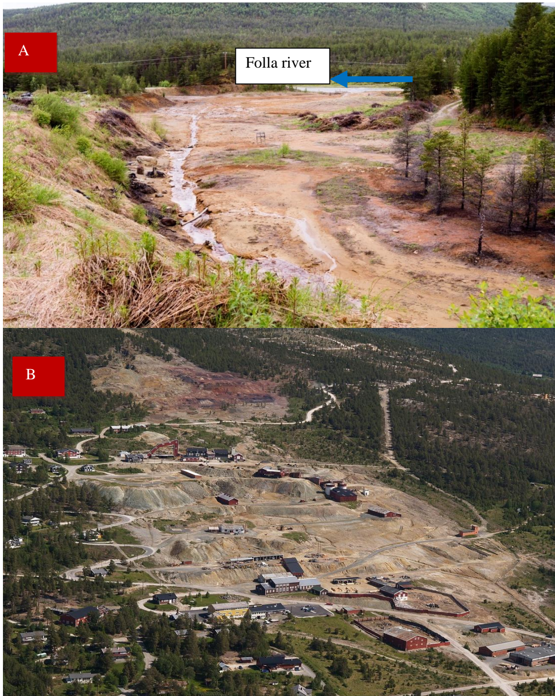
Fig 2.7 The acid mine drainage discharging to Folla river (A) and bird eye view of Folldal Main mine area: production buildings and workers cottages (B) (Folldal Gruver, 2015).
