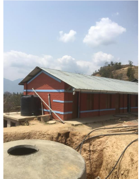
Figure 34. The newly built water storage tank, with a nearby building that easily can exploit the potential for rainwater harvesting. Photo Ø.M.
