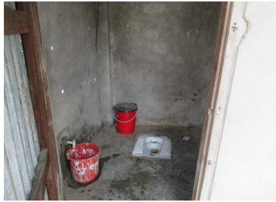
Figure 11. Inside the girls and teachers toilet. Photo Ø.M.
