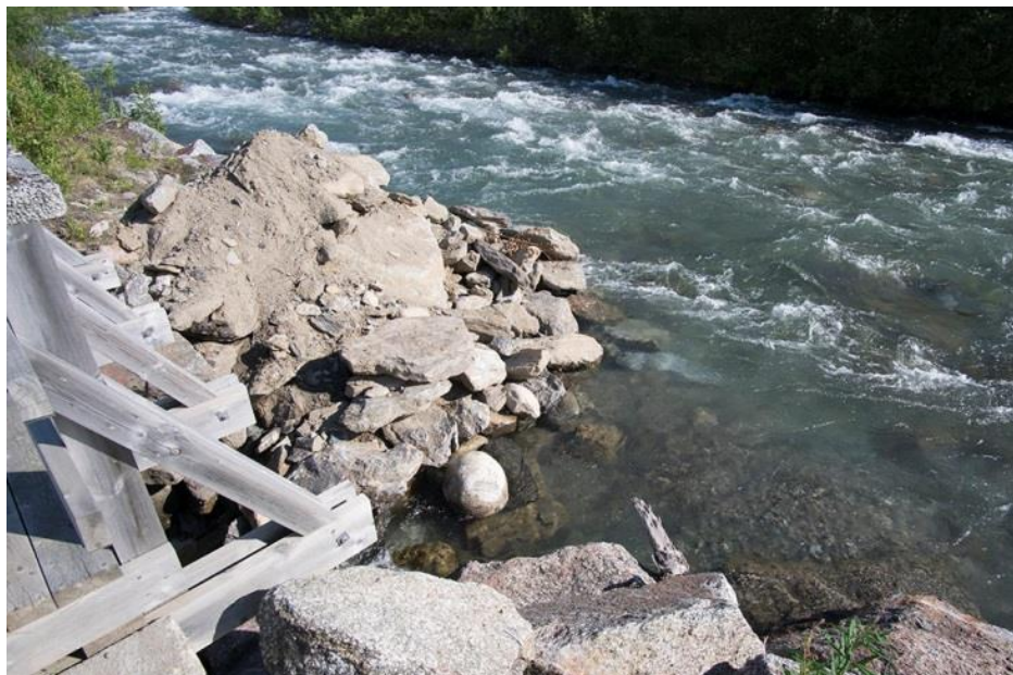
Figure 31. Boulders blocking the intake to Budalsfaret, due to fear of a destructive flood.
