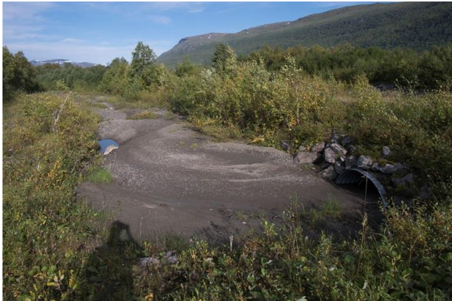
Figure 25. The reopened tributary at Gåsodden, where the intake causes accumulation of sand, gravel and cobble.
