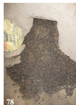
Figure 76: Traditional dry toilet with ash as an amendment and a box for non-degradable waste
