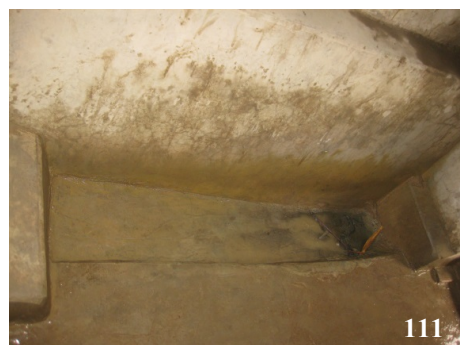
Figure 111: Cemented urinal ditch with clogged drain
