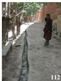
Figure 111: Cemented urinal ditch with clogged drain
