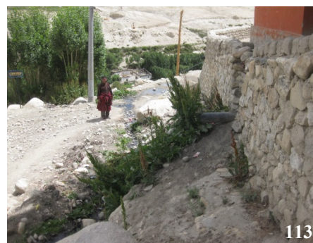
Figure 112: Channel leading urine and graywater along the city wall to the northwestern corner of town
