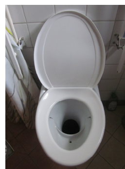
Figure 171: Urine-diverting toilet seat (here in Tingvall, Sweden)
