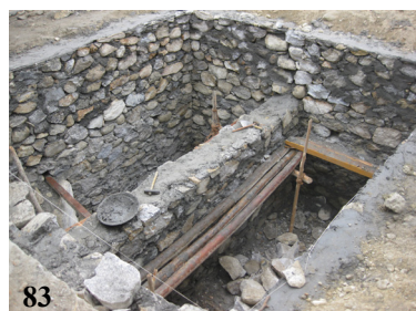
Figure 83: Leaching cesspool under construction at a private school in Lo Manthang
