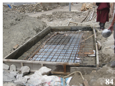
Figure 83: Leaching cesspool under construction at a private school in Lo Manthang
