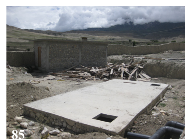
Figure 83: Leaching cesspool under construction at a private school in Lo Manthang
