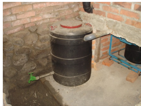
Figure 150: Urine storage barrel with outlet tap (ENPHO, n.d.-e)
