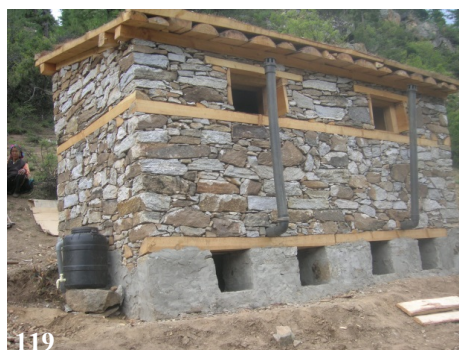
Figure 117: Compost toilet developed in Norway with solar ventilation and dehydration mechanism
