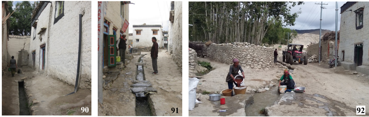
Figure 90: Channel that used to be Lo Manthang's drinking water source; a domestic graywater pipe leading directly into the channel
