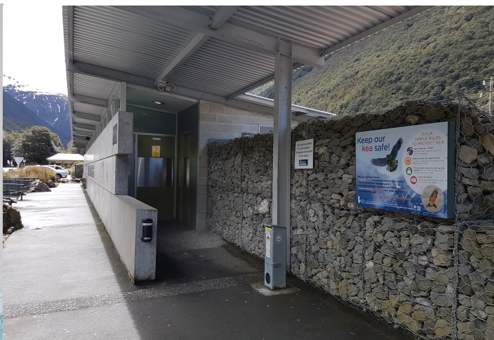
Figure 9: Sign at the carpark/public toilets, same as at the Viaduct
