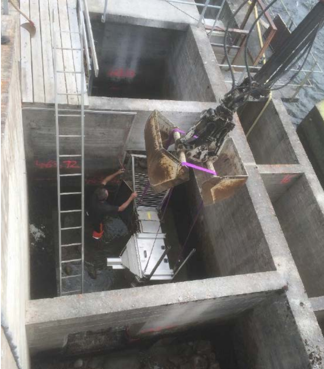
Figure 7 - The VAKI Riverwatcher gets lowered into chamber nr.15 of the fishway on the 16 th of June, 2016 (Taugbøl 2016).
