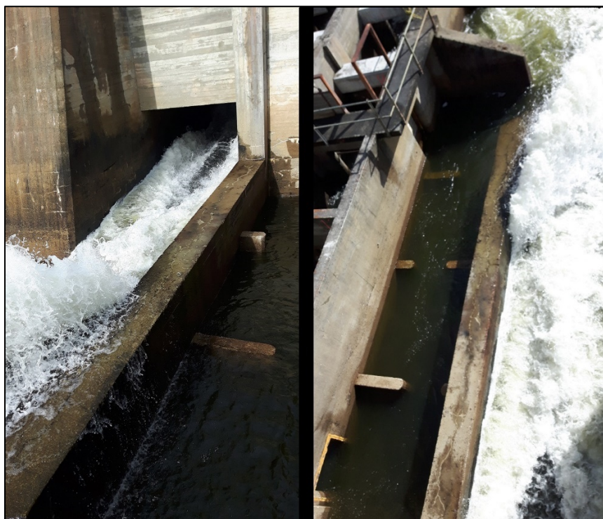
Figure 4 - These two pictures illustrates how it looks around the fishway entrance when 15 m 3 /s of water is led through the tap-spillway. The tap spillway opening is seen in the left picture, while the fishway entrance is seen in the right picture. The water velocity in the lower sections of the fishway is low compared to the flow released from the tap spillway. Picture taken April 10, 2017.
