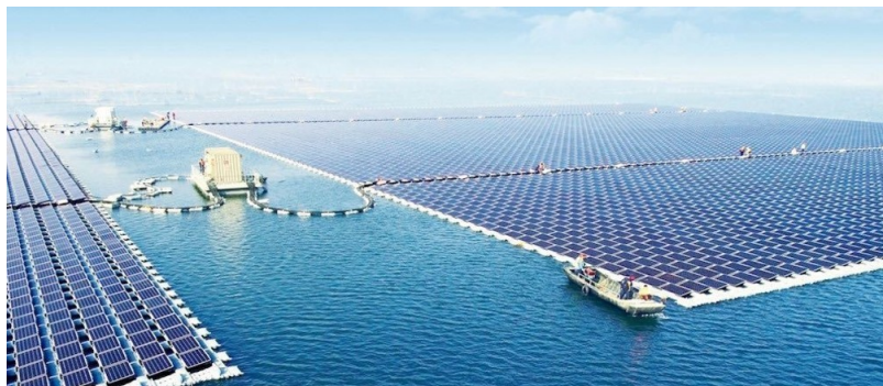
Figure 2.7: Floating solar power plant in Huainan, China (Brandon, 2017)
