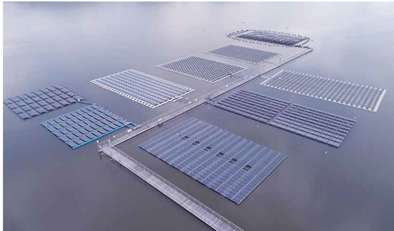
Figure 2.9: Testbed in Singapore with 10 installations of floating PV (Reindl, 2018)
