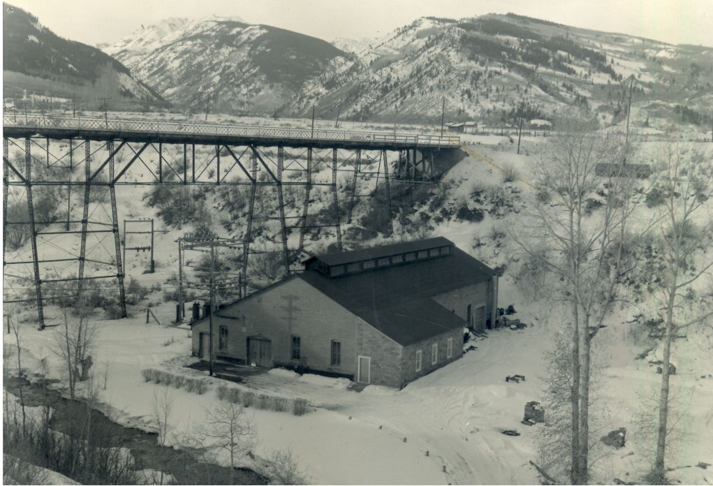
The old hydroelectric plant next to Castle Creek. Photo Credit: Aspen Historical Society.
