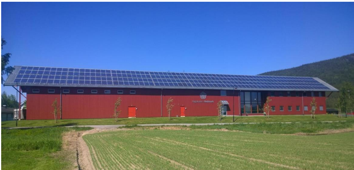
Figure 3.1. The PV array on the roof of the barn at Campus Evenstad. From [32].
