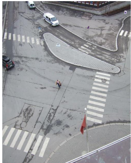
Figure 12. St. Olavs plass before redesign approx. 2005, photo: ACK Architects
