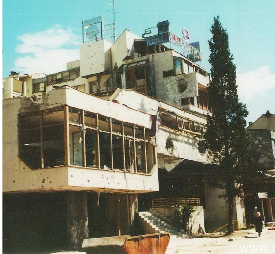
Figure 17: Destroyed commercial buildings close to the Old Town. (Cidom, 2017.)
