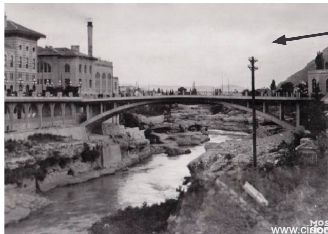
Figure 14: The remade bridge in concrete, crossing from the new city centre to Musala Square. (Cidom, 2017.)
