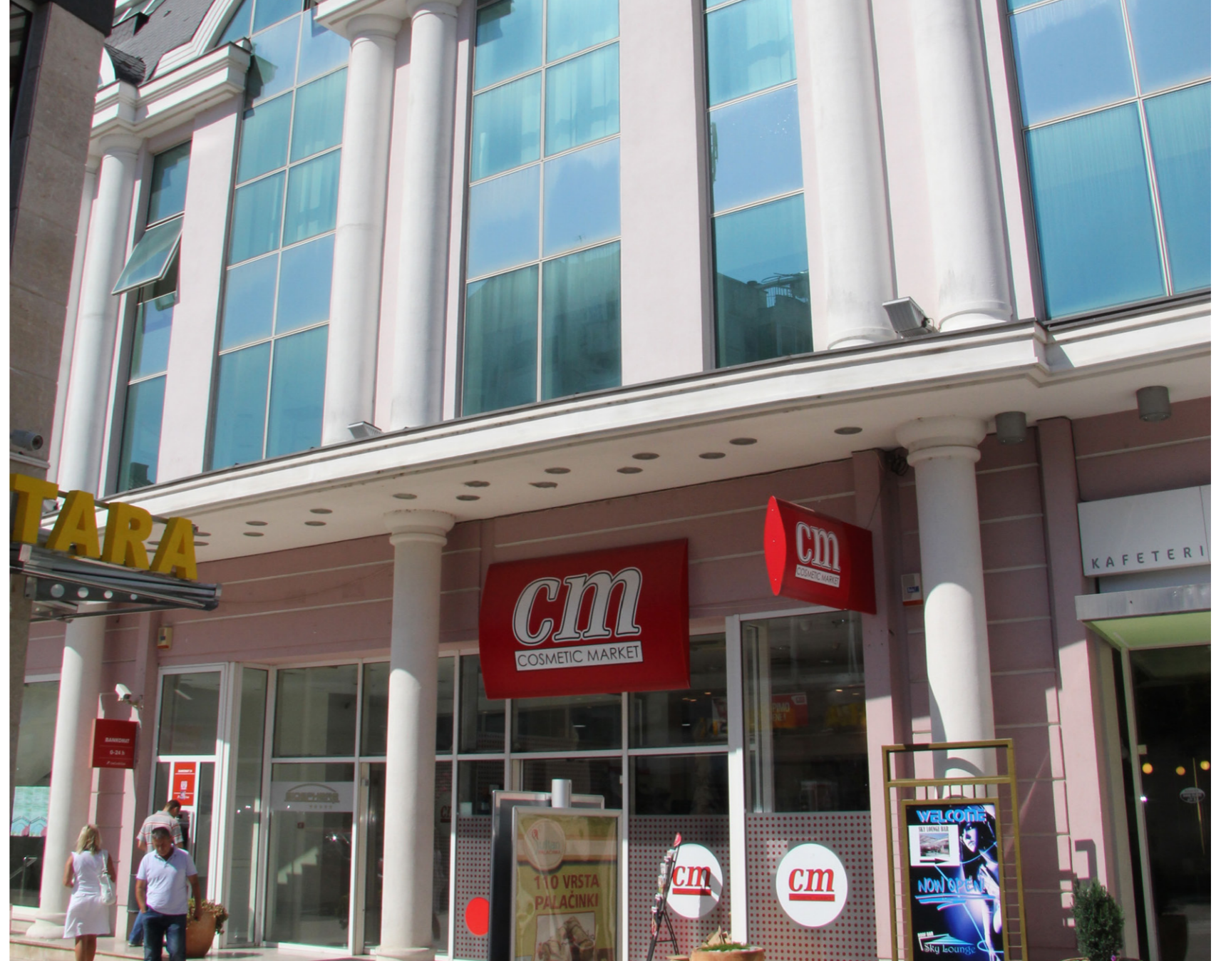
Figure 120: Commercial building located somewhere closeby to the old town. (Brkan, 2017)
