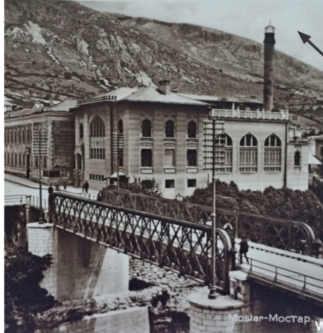
Figure 13: The original steel bridge that crosses to the Musala Square. (Cidom, 2017.)
