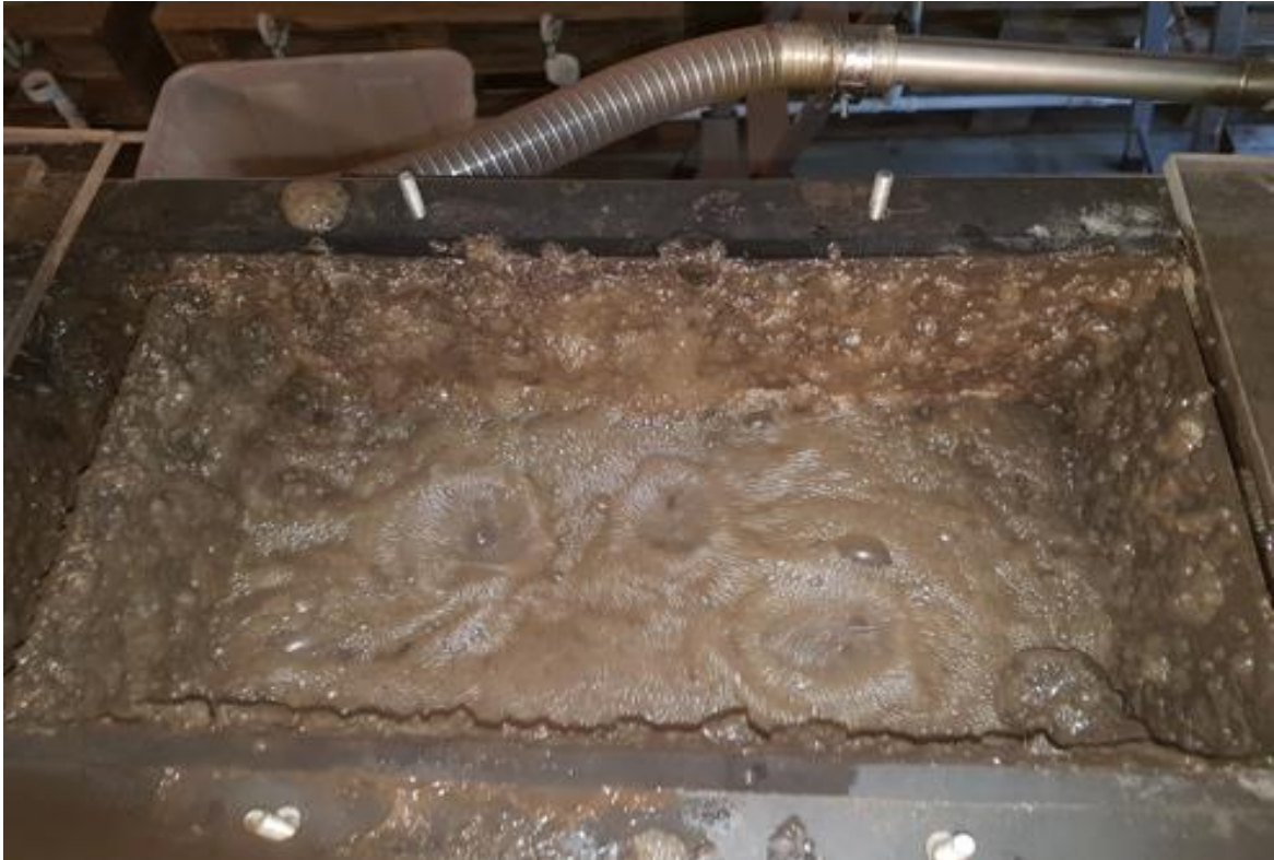
Figure 22: Foaming in the separation chamber
