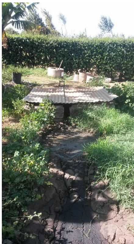
Photo 9: The fixed dome biogas system showing the inlet, the digester and the slurry outlet. Photo: Stephen Ngugi Wamwea.
