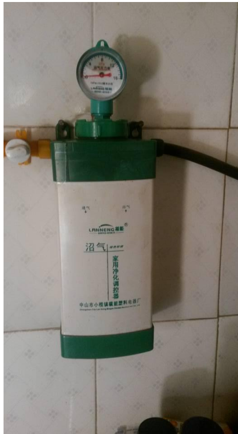
Photo 12: The biogas desulphurizer showing the manometer gauge. Photo Stephen Ngugi Wamwea.
