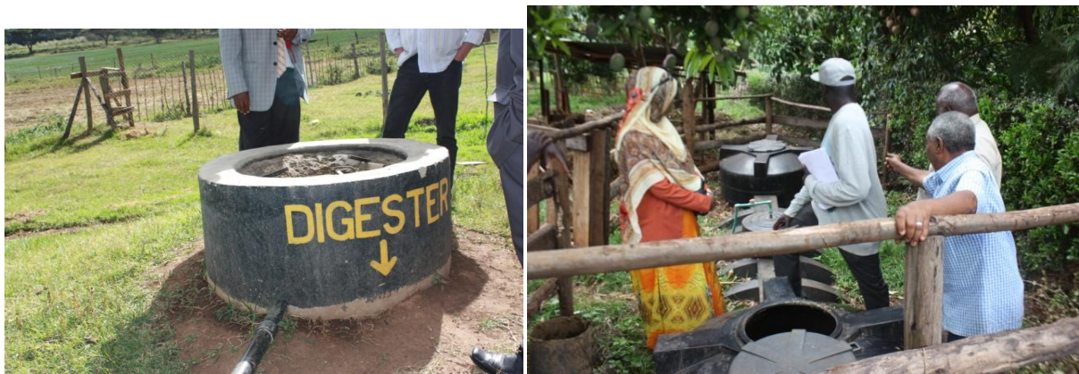
Photo 3: The Biogas digesters. Left: Brick and concrete digester buried in the ground. Right: Prefabricated plastic digester buried halfway in the ground. Photo: (Wamwea, 2010).
