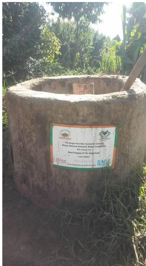
Photo 4: The inlet tank. Photo: Stephen Ngugi Wamwea.
