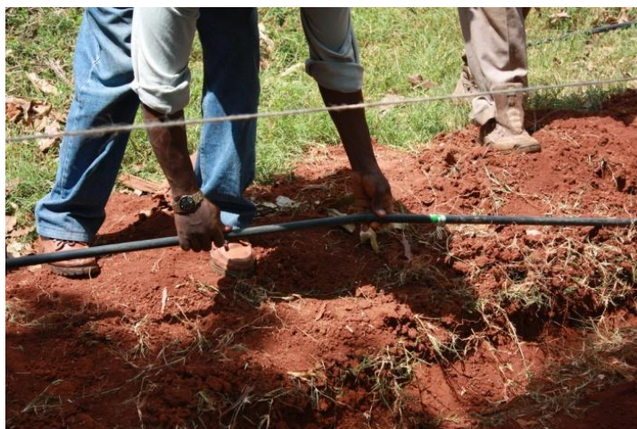
Photo 5: Laying the pipes in the trench. Photo: (Wamwea, 2010).
