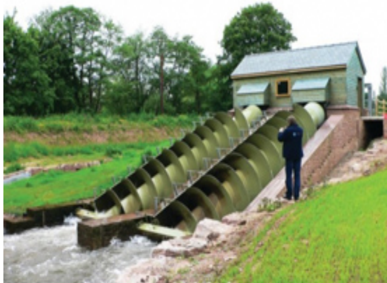
Figure 4: Small Hydro-power plant at initial stage of nineteenth century. Source: hydropower in New-York; NYS department of Environmental conservation.
