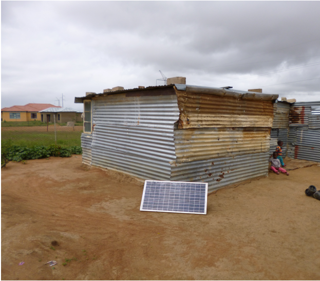
Figure 4-4: Typical shed with a PV module from the SHS in Nobody New Stand
