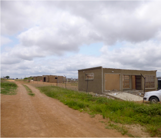
Figure 4-3: Typical small house and road infrastructure in Nobody New Stand
