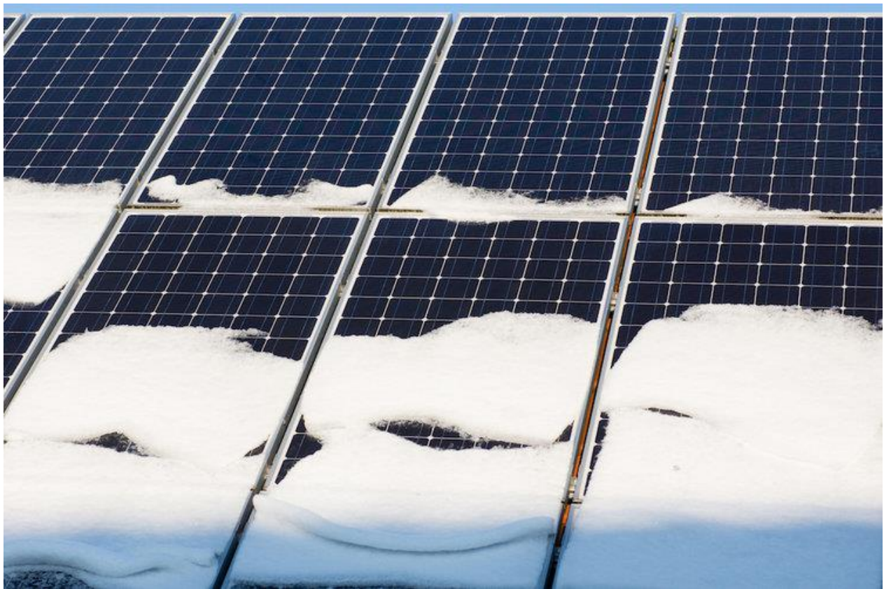
Figure 15. Partially snow covered modules. (Drews 2017)
