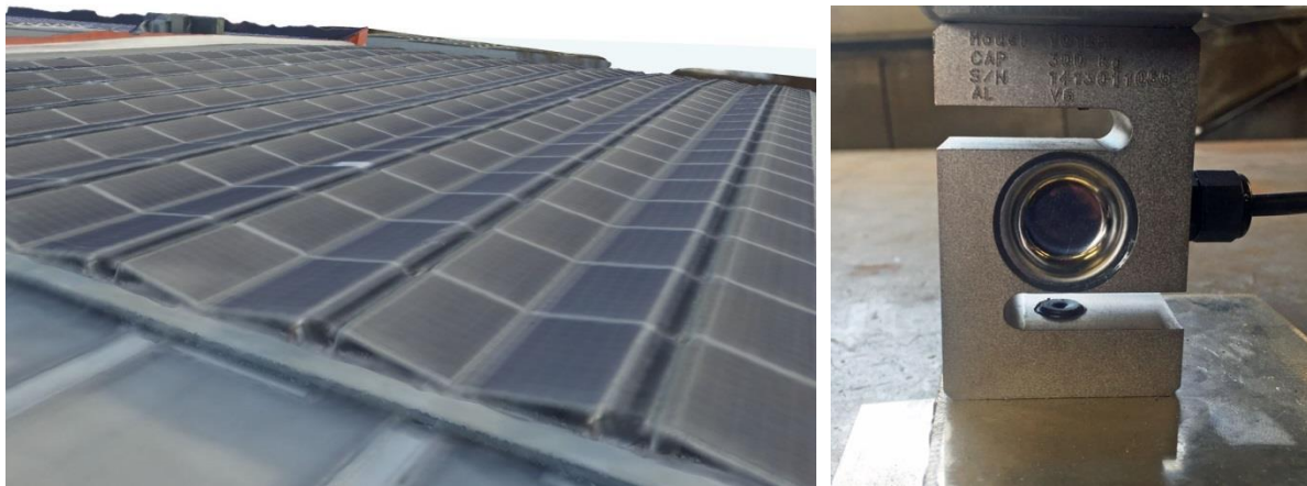
Figure 14. The left picture shows how the Weight Watcher system is assembled. A large part of the roof surface is covered with modules. The modules have a low angle tilt preventing the snow from sliding off. The picture is a 3D model of the roof made from drone pictures produced in this thesis. The right picture shows the load sensor installed at the frame of the modules.
