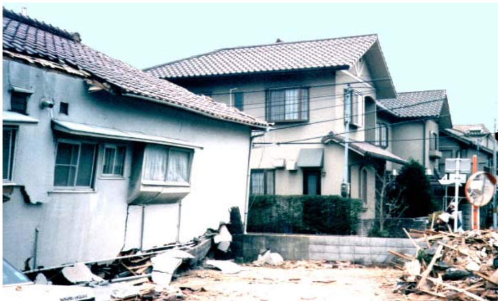
Figure 1: Three undamaged modern wood frame buildings (background) next to an older building (foreground) whose ground floor has collapsed completely.
