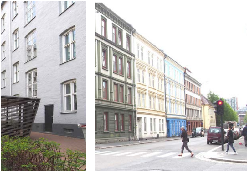
Figure 5-4 Overall photos of Resident-Managed Courtyard
