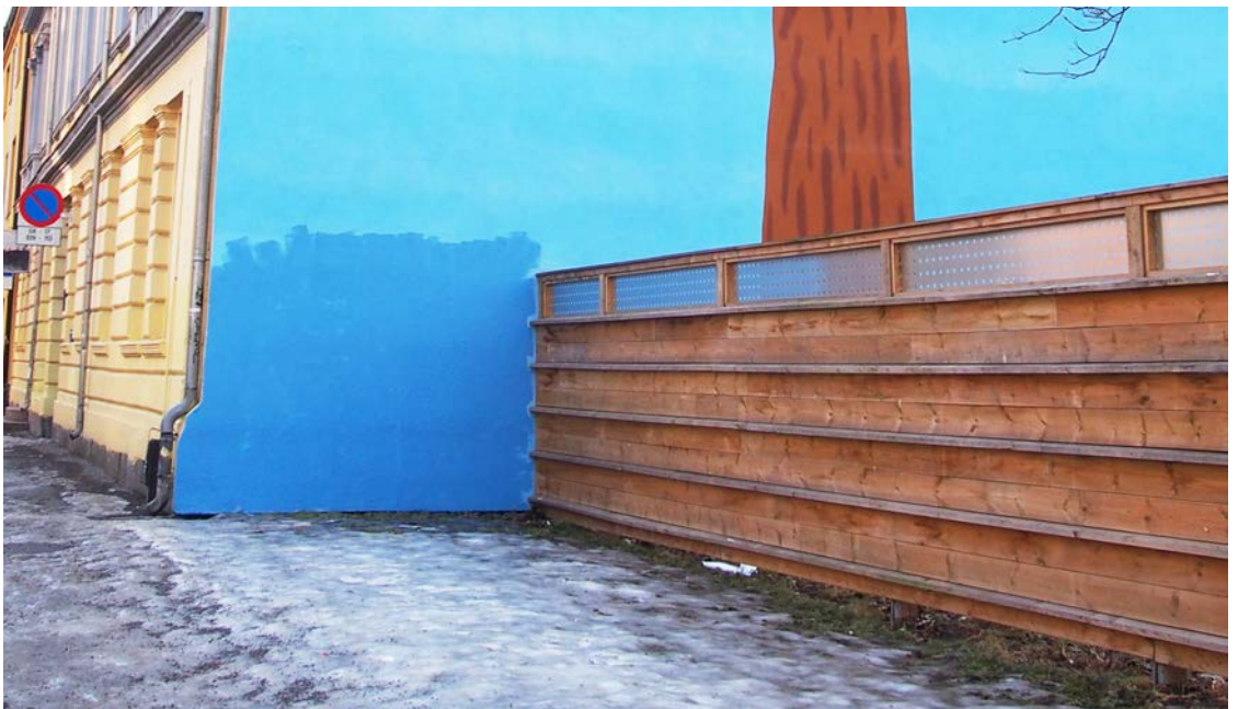
Figure 7-9 Boundaries like fences can catch litter and screen engagement activities from informal surveillance, as in this fence and graffiti-targeted wall surface at Publicly-Managed Social Housing.
