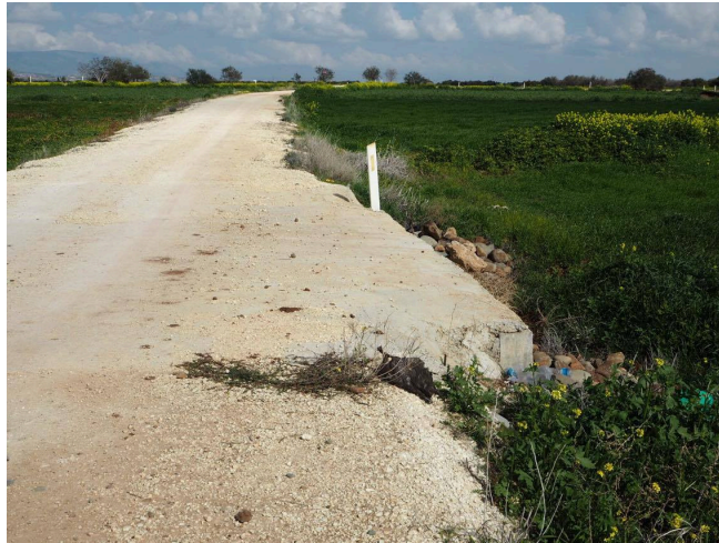
Figure 34: As a result of land consolidation gravel roads are constructed with a slope for proper drainage.
