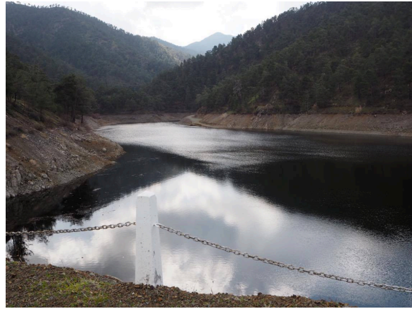
Figure 30: The Xyliatos Dam providing water for the inhabitants as part of the land consolidation scheme.
