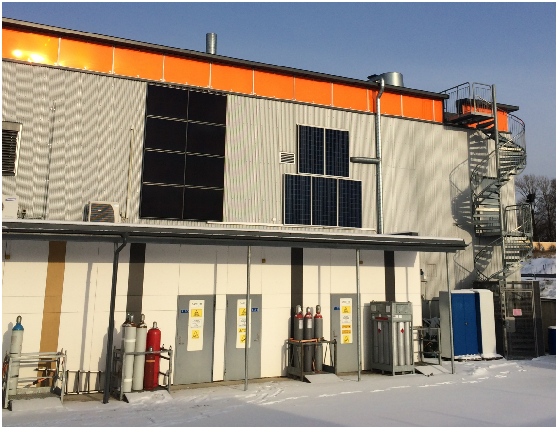
Figure 33: Picture of the two PV systems mounted on the roof on Kjeller. The picture was taken on November 9, 2016 at 12.30. To the left is the thin-film system and the silicon-based system is to the right.
