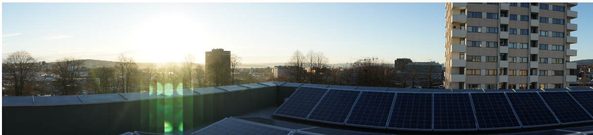
Figure 27: Illustrating the south-west corner of the building and one of the main sources for shading on the system. The picture is taken December 1, 2016 at 14.15. At this time a year the Sun sets before it reaches the building to the right.
