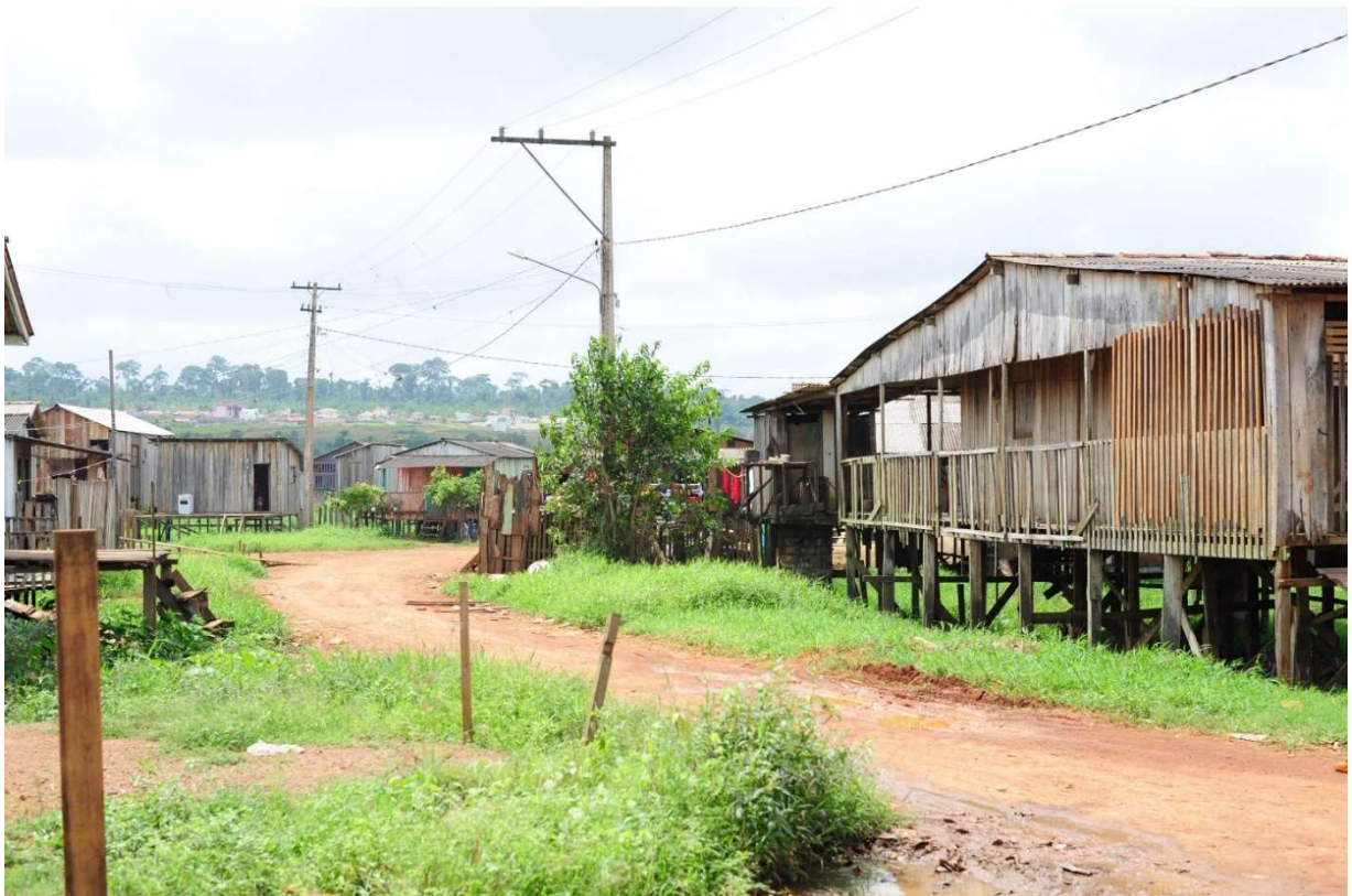
Fig.10 Boa Esperança district in Altamira before demolition (2013) Photo: Tove Heiskel
