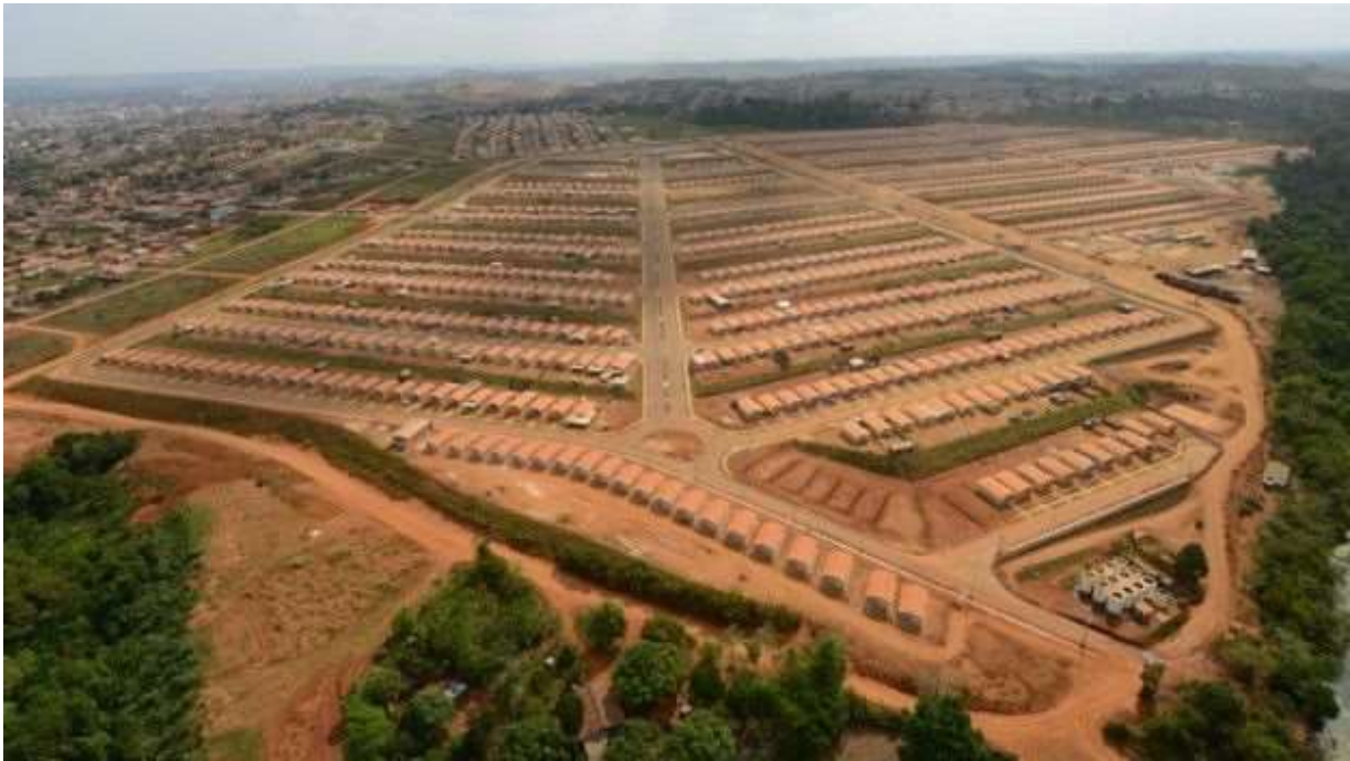
Fig. 11. Jatobá, where housing for 1,100 families was constructed. Photo: Regina Santos
