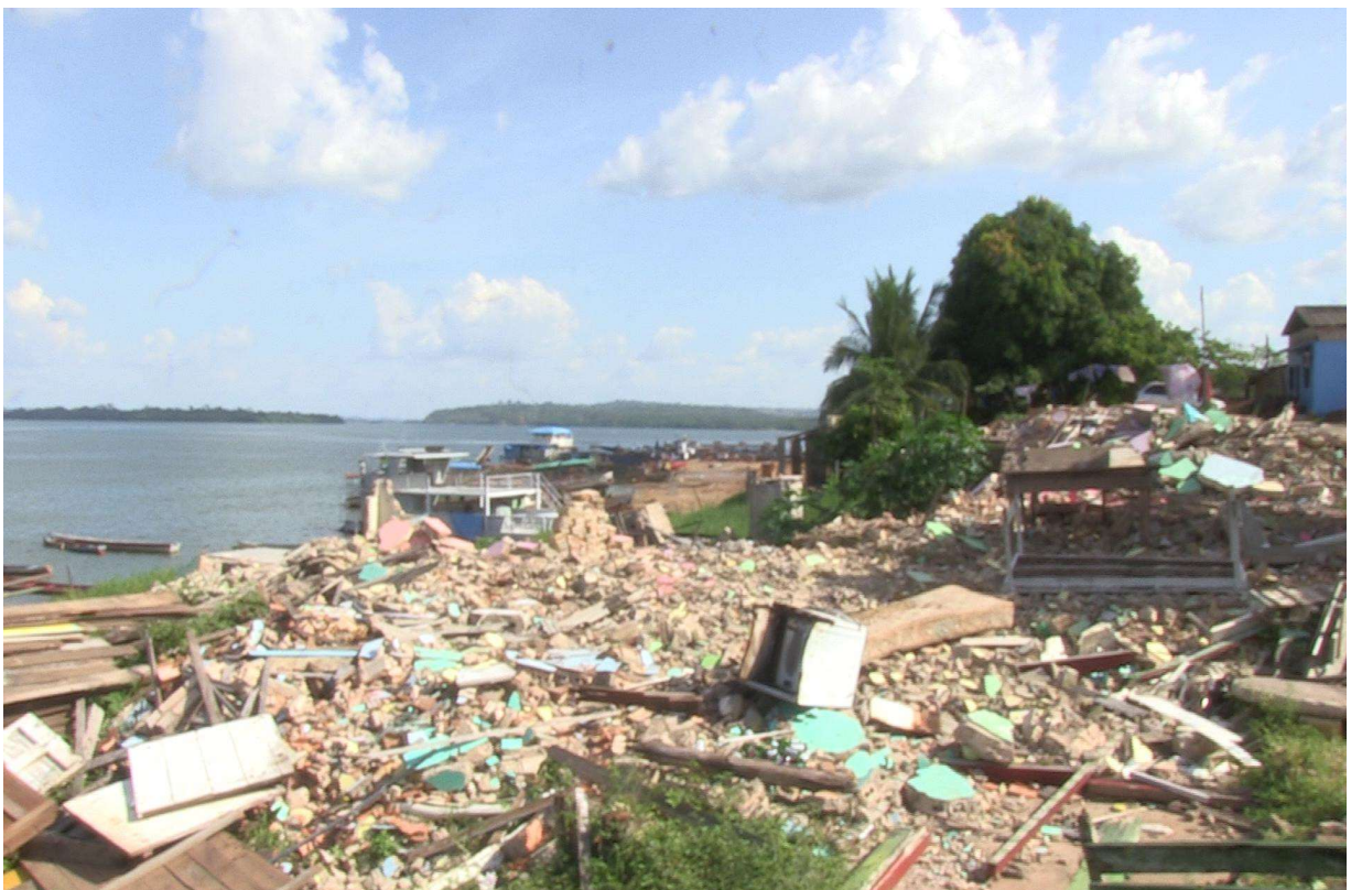
Fig.8. Demolished houses by the riverside in Altamira city (2015). Stills from video footage: Tove Heiskel
