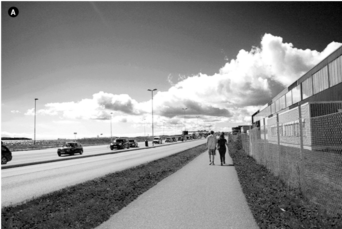
Fig.47: One of the few pathways for bicyclists and pedestrians in the ferry terminal area
