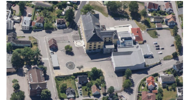
Fig.79: Orthophoto, statement building
