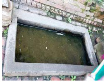
Underground cement tank
