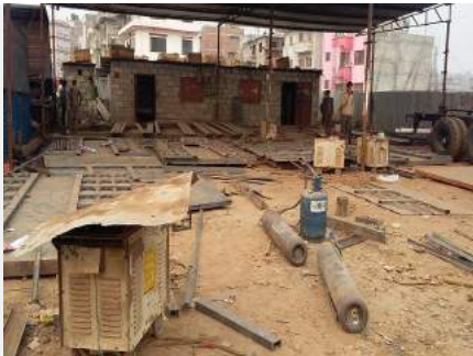
Metal repairing centre
