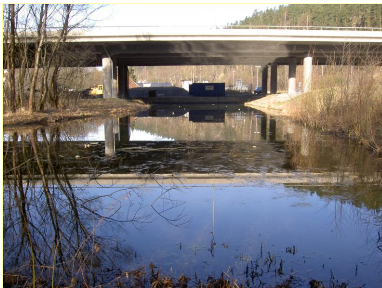
Figure 11. Picture showing the bridge on E6 crossing the Skullerud sedimentation pond. The picture is taken from the pond outlet towards the pond inlet. The blue steel container in back of the picture was used as a field laboratory during the experiment presented in Paper III.
