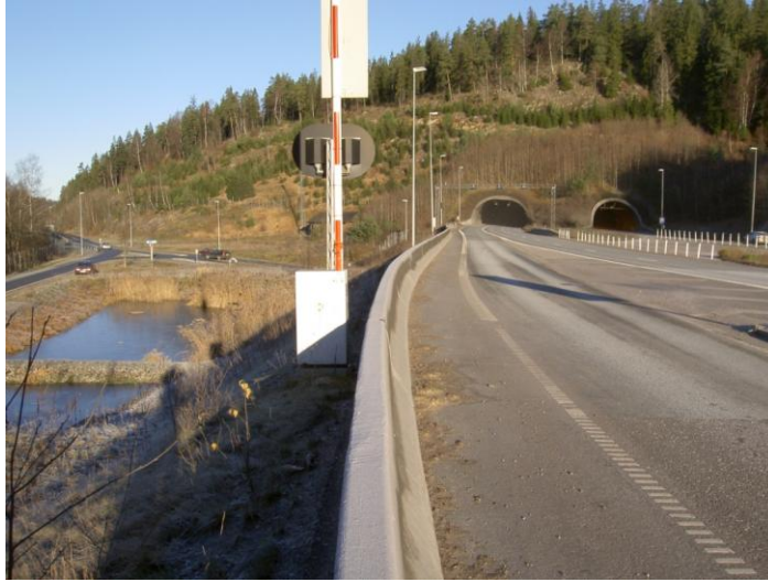
Figure 10. The Vassum junction with the Nordby tunnel to the right hand side and the sedimentation pond to the left hand side. The pond inlet is in front of the picture, while the pond outlet is in the back.
