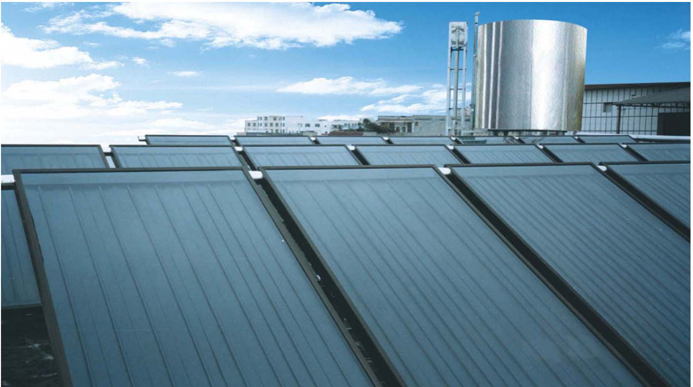
Fig. 2.3.: Figuren viser flere plane solfangerer. Kilde: http://gogreenheatsolutions.co.za/?q=project-type/solar-water-heating/flat-plate-collector
