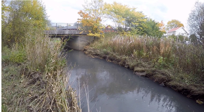
Figure 22 – Vigga downstream after the release of untreated pit water.
