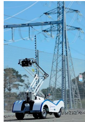
Figure 2.13: Transpowers Substation Robot with its arm raised for a better camera view. Photo by permission of Transpower New Zealand.
