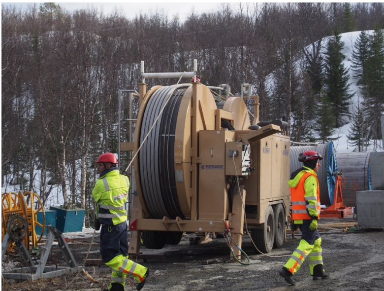
Figure 0.2: Photo of a puller for large cables like Hubro.
