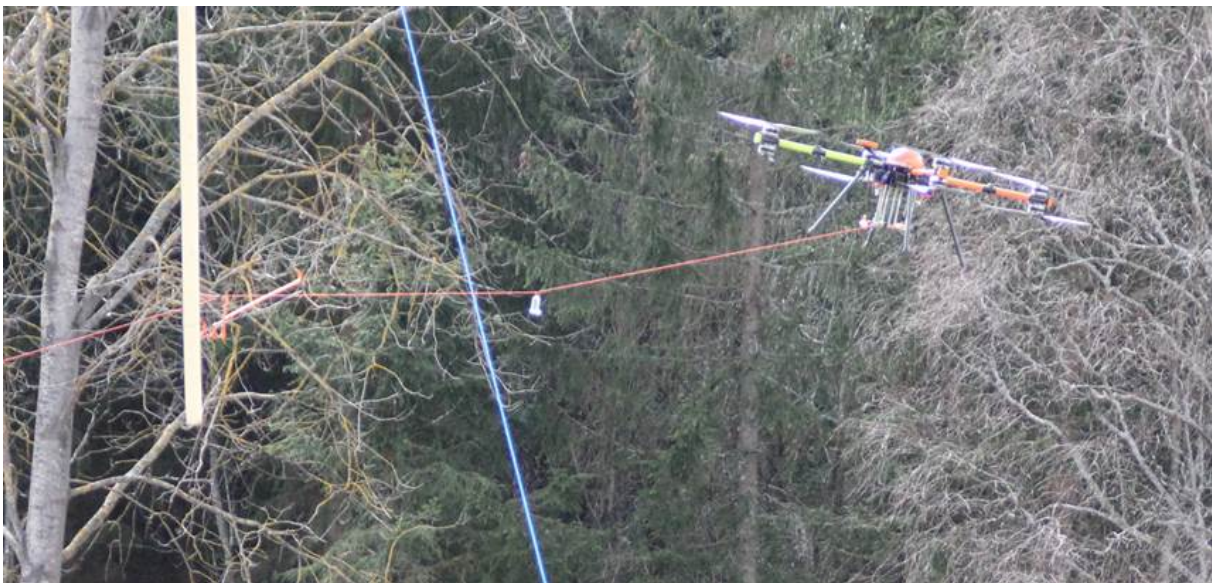
Figure 2.8: UAV placing a pilot line in a temporary tower. Photo with permission by Knut Stabell, captured on the 27th of april 2016 at Sørkedalen during the testing of UAVs to pull pilot lines. UAV operator was Nordic Unmanned.
