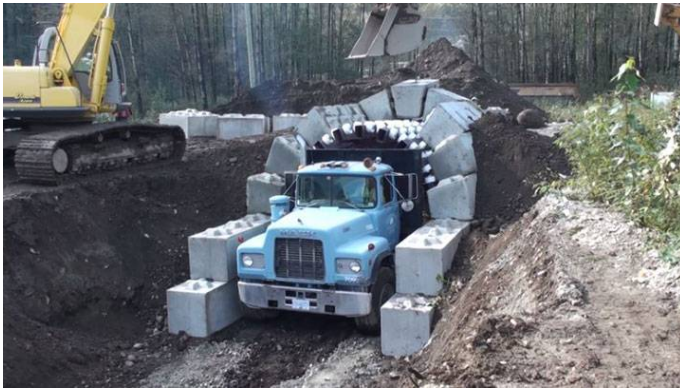
Figure 0.1: Zipper truck for building of small tunnels. Photo by permission of Lock-Block
