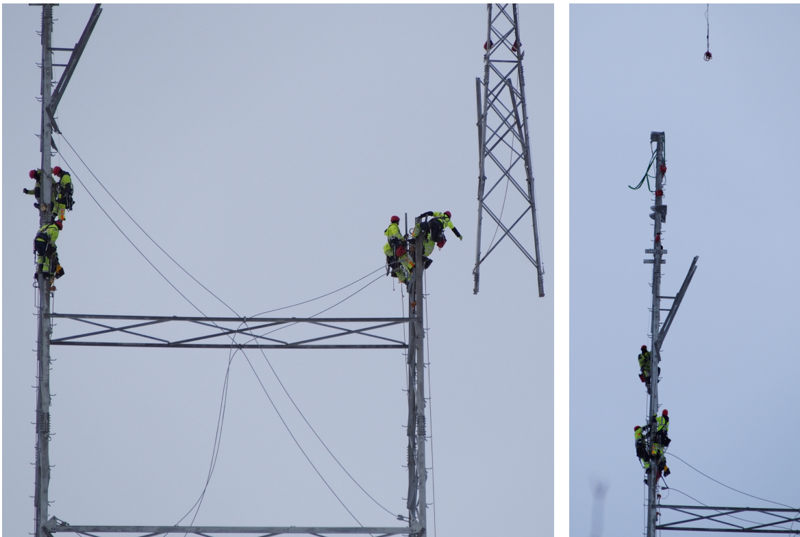
Figure 3.8:Left: An assembler reach out to grab the incoming cargo. This piece is then mounted on top of there the assembler is located.
