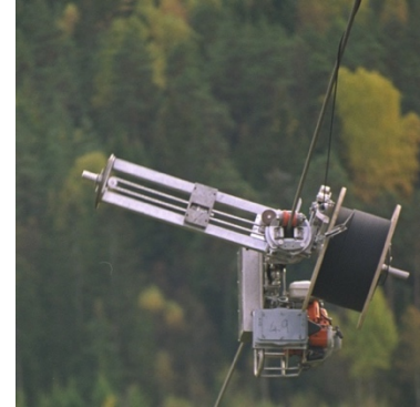
Figure 2.2: SkyWrap® wrapping a fiber optic cable around a conductor. Photo by permission of AFL
