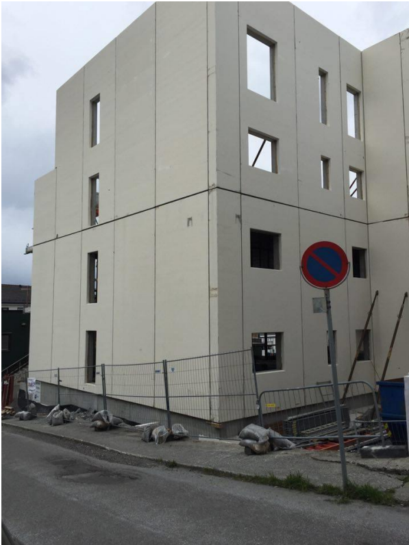
Figure B - 2: Picture 2 from the assembly of the construction
