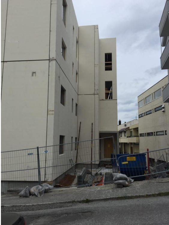
Figure B - 1: Picture 1 from the assembly of the construction
