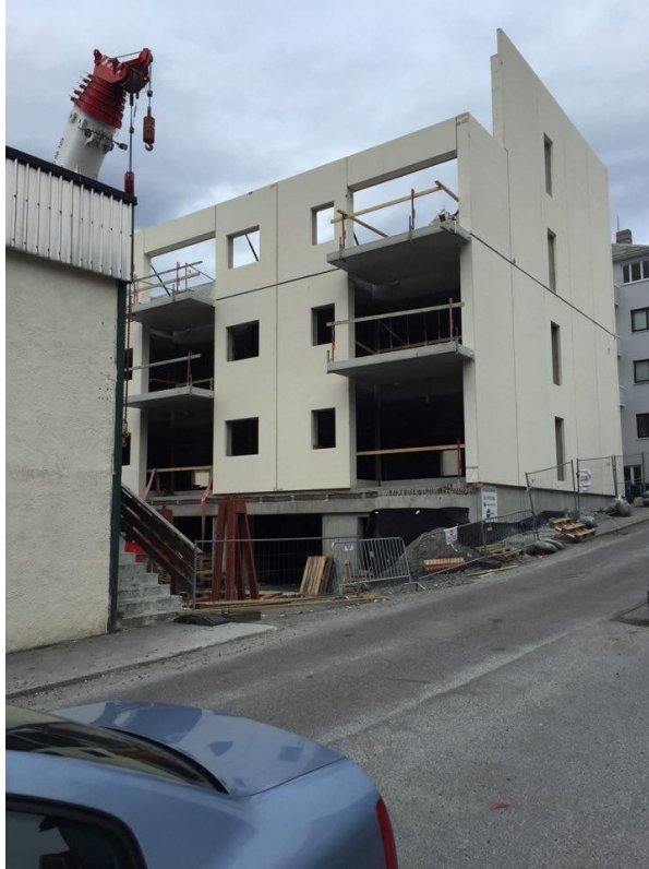
Figure B - 3: Picture 3 from the assembly of the construction
