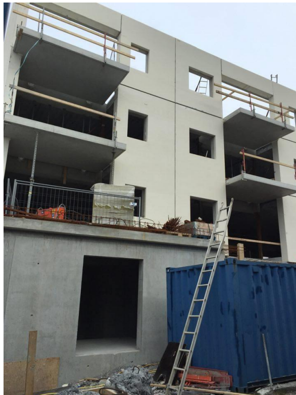
Figure B - 4: Picture 4 from the assembly of the construction
