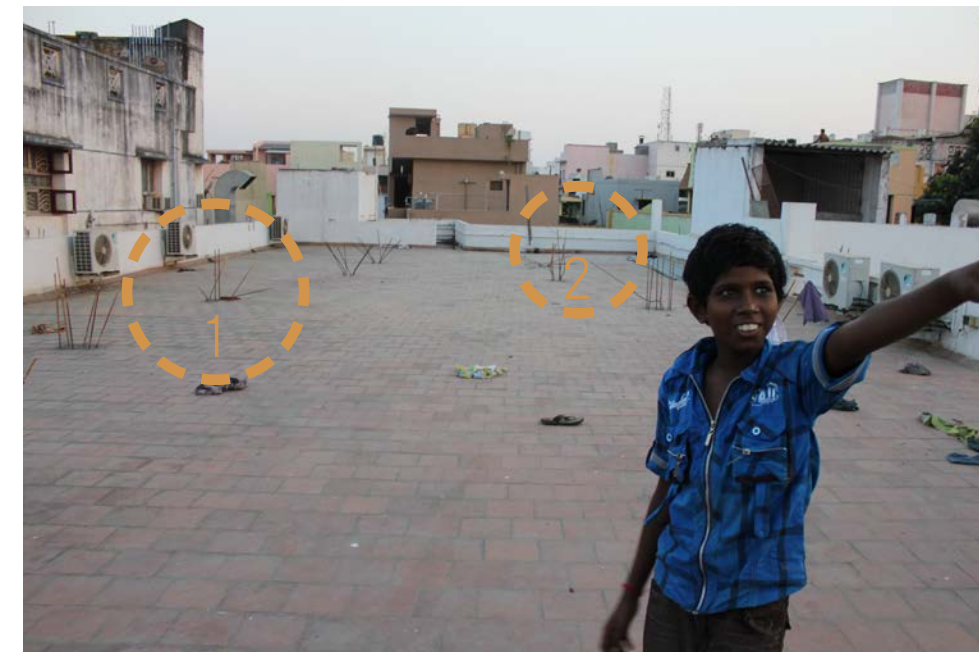
1. Steel poles sticking up from the roof. 2. Low masonry wall, easy to climb over.
