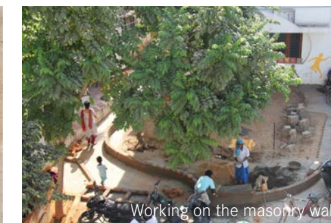
Working on the masonry wall.
