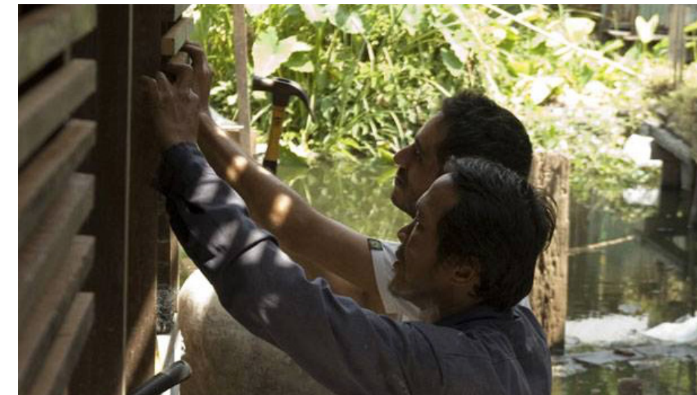
Fig 9: The community working together on the Ole Market Library project.
