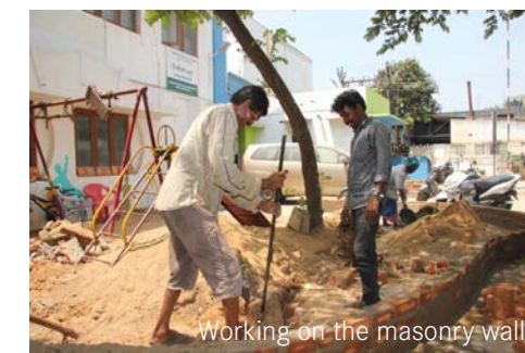
Working on the masonry wall.
