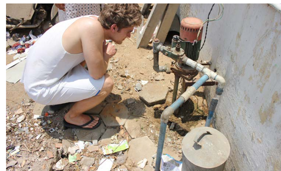
Water system seems to be in good shape.
