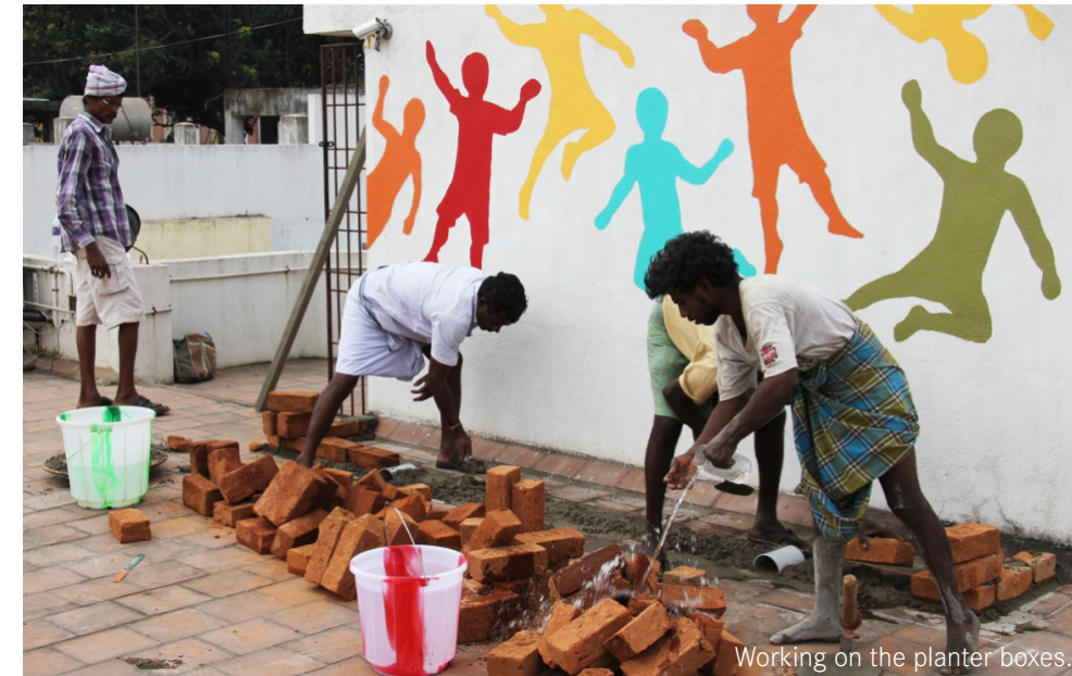
Working on the planter boxes.
