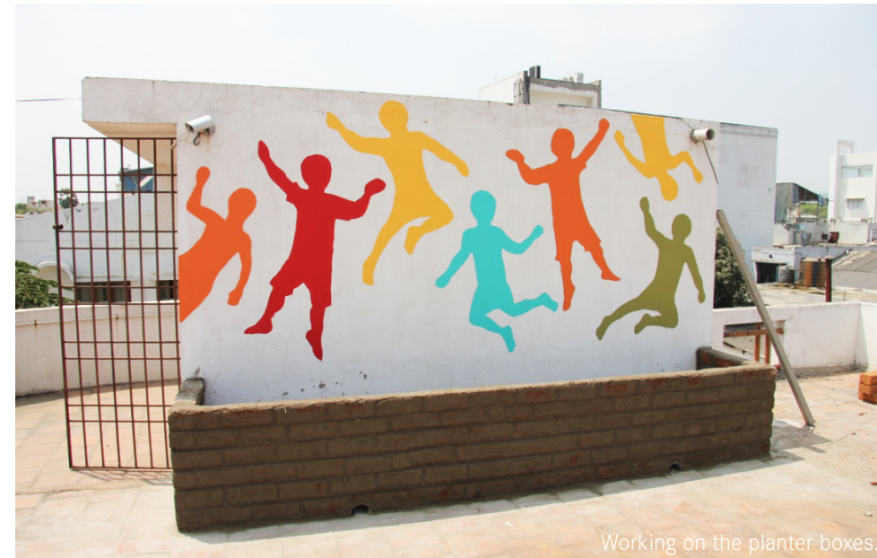
Working on the planter boxes.
