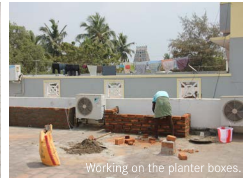
Working on the planter boxes.
