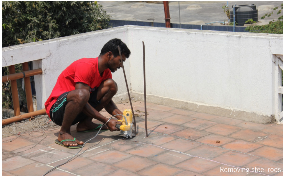
Removing steel rods.
