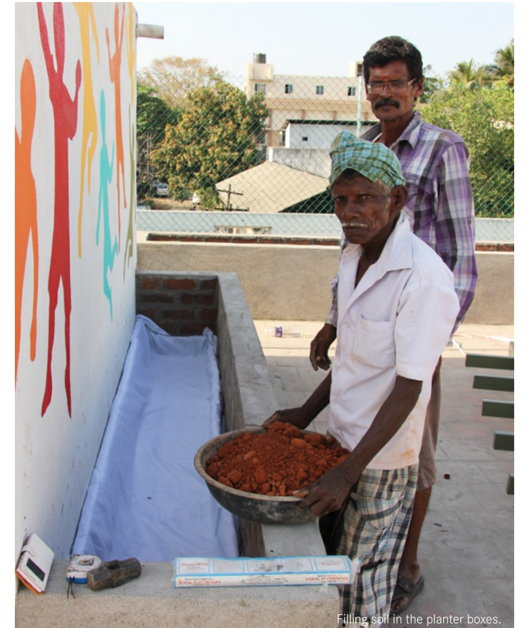
Filling soil in the planter boxes.
