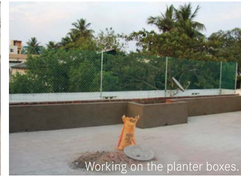
Working on the planter boxes.
