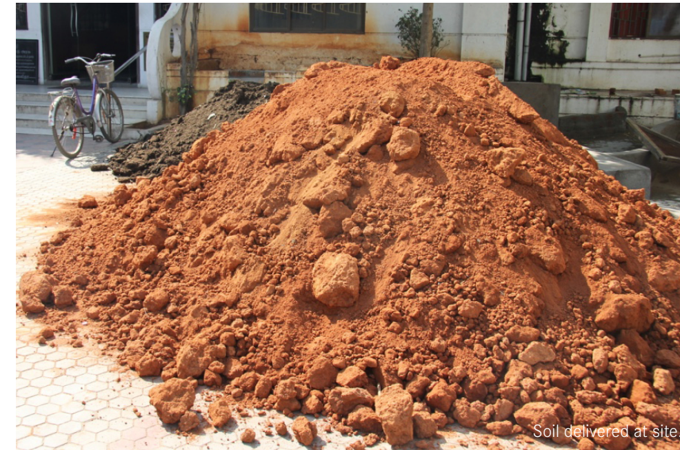
Soil delivered at site.
