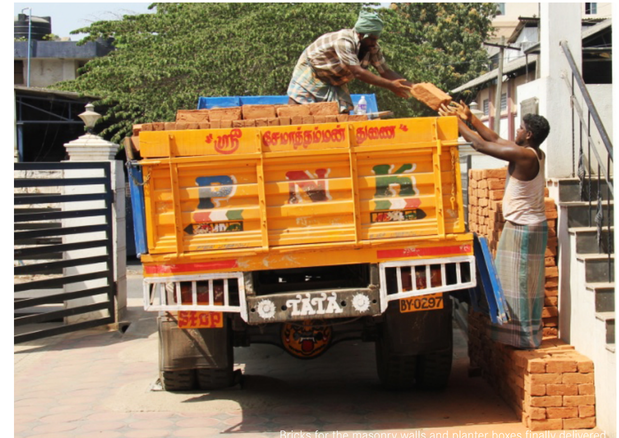
Bricks for the masonry walls and planter boxes finally delivered.
