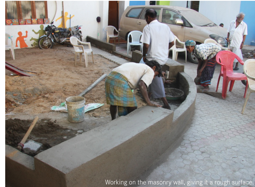
Working on the masonry wall, giving it a rough surface.
