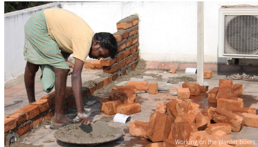
Working on the planter boxes.
