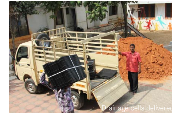
Drainage cells delivered.
