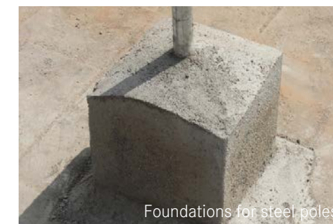
Foundations for steel poles.
