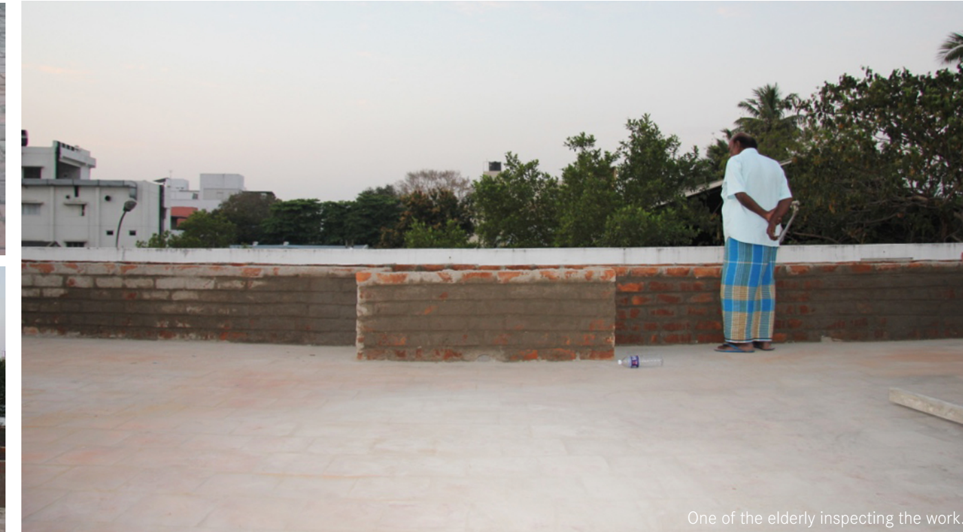
One of the elderly inspecting the work.
