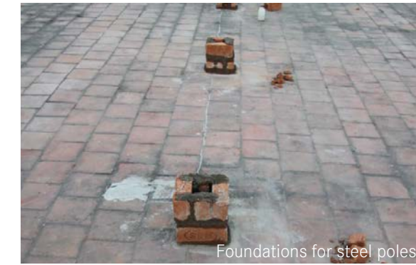
Foundations for steel poles.
