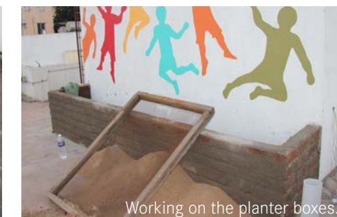
Working on the planter boxes.
