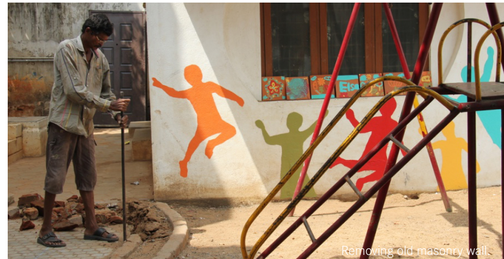
Removing old masonry walls.
