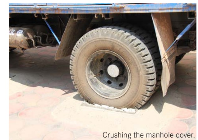
Crushing the manhole cover.
