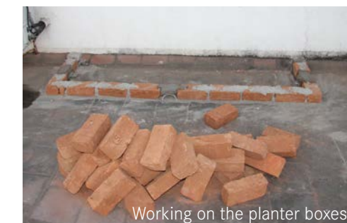
Working on the planter boxes.
