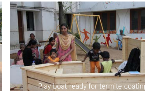
Play boat ready for termite coating.
