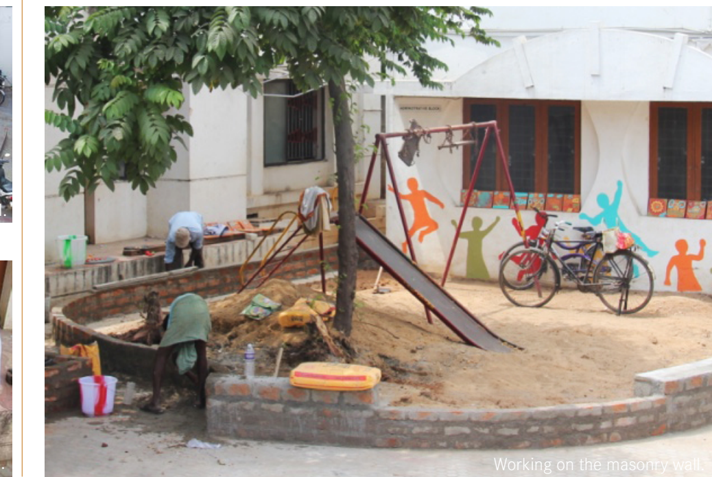
Working on the masonry wall.
