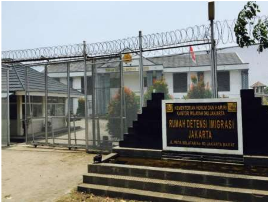
Figure 4. Detention center from outside
