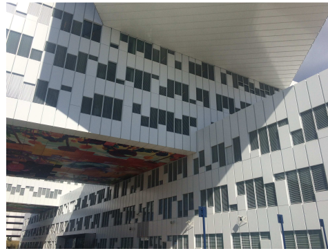
Figur 11: Overlapping mellom lameller, Statoil. Kilde: C.Blix
