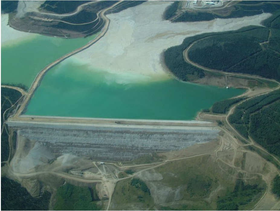
Photo: Earthen tailings impoundment dam at Fort Knox gold mine in Alaska. This tailings impoundment dam at the Fort Knox gold mine in Alaska is a common method of storing mining waste forever. (Photo retrieved: http://www.groundtruthtrekking.org/photo/typical-mine-tailings-dam/ )
