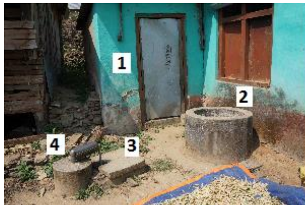
Figure 34 – A toilet (1) connected to biogas reactor including a grinder (2) for addition of manure and organic waste, a lid (3), and a gas pipe (4) connected to household stove in Chakratirtha (photo taken by the authors)
