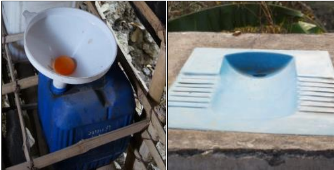
Figure 43 – Simple urine diversion technology. Male jerry can urinal (left) and female urine pan (right) to be piped into a jerry can below (Photo taken by authors)
