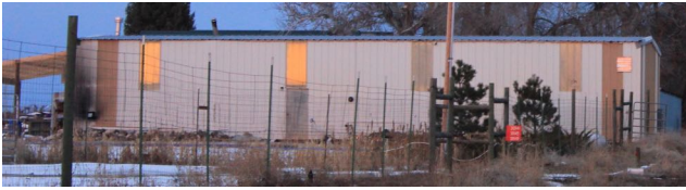
Figure 10 Indoor grow facility
