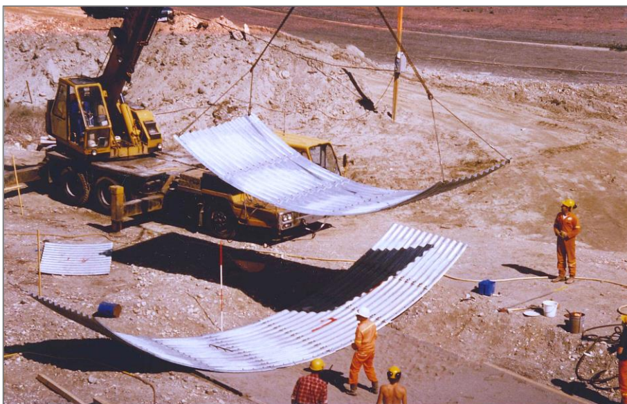
Figure 2.7. The base structure lifted with crane into the pre-formed soil (Vaslestad 1985).
