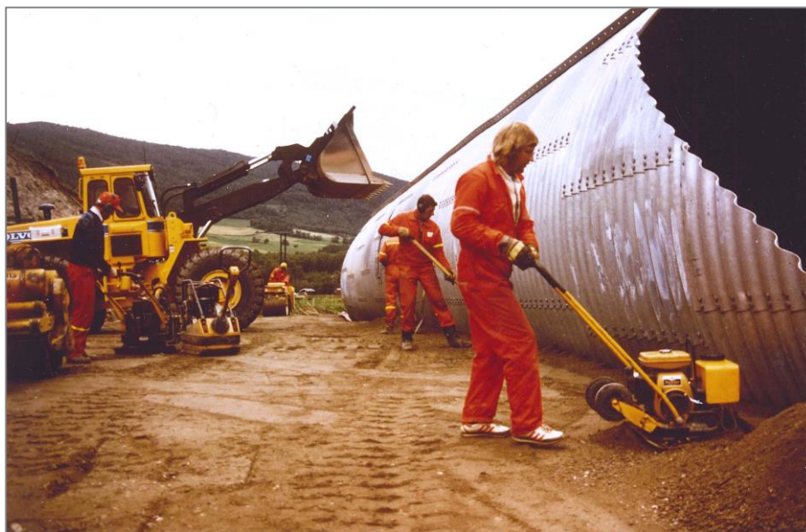
Figure 2.10. Compaction of backfill with manual labour and a plate compacter (Vaslestad 1985).
