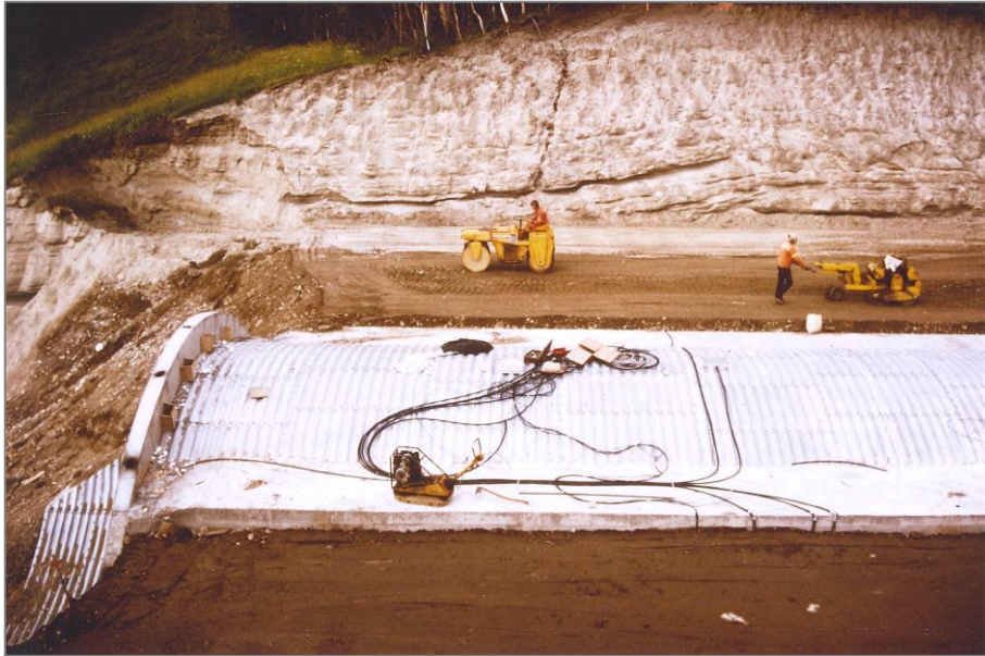
Figure 2.11. Compaction of backfill with a vibration roller (Vaslestad 1985).
