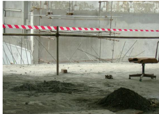
soft and hard barricated is in place to prevent fall hazards
