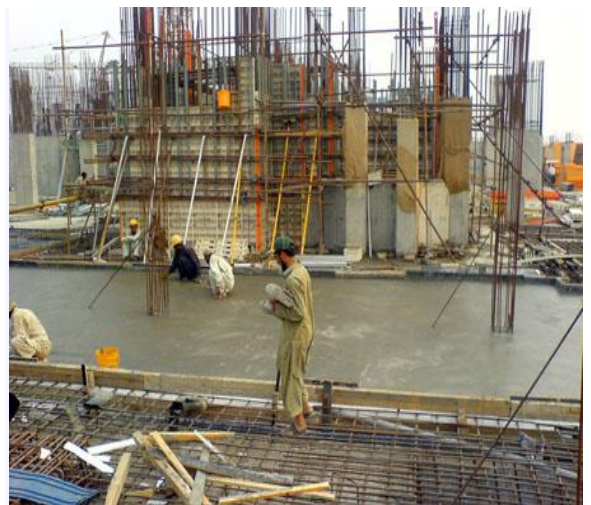
Slab casting at the basement level
