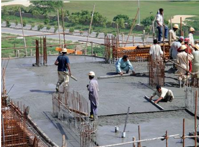
Concrete pouring on top floor of the building
