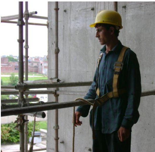
workers are provided with safety belts and helmets
