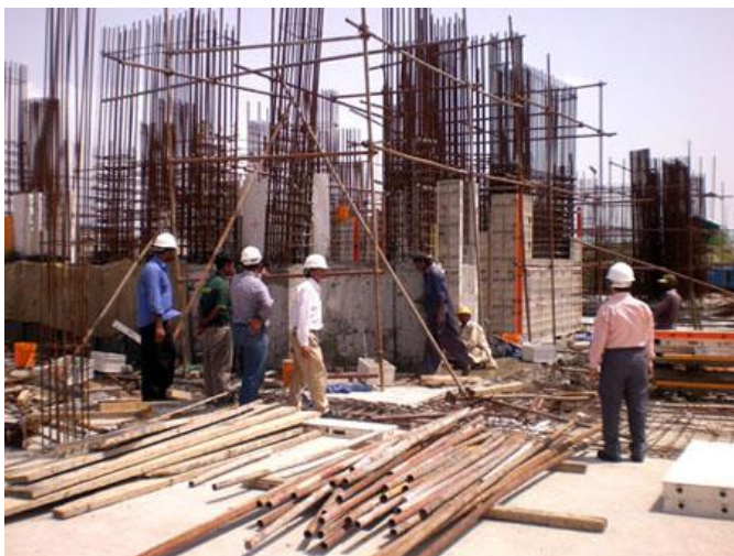
Installation of reinforcement to shear walls and columns
