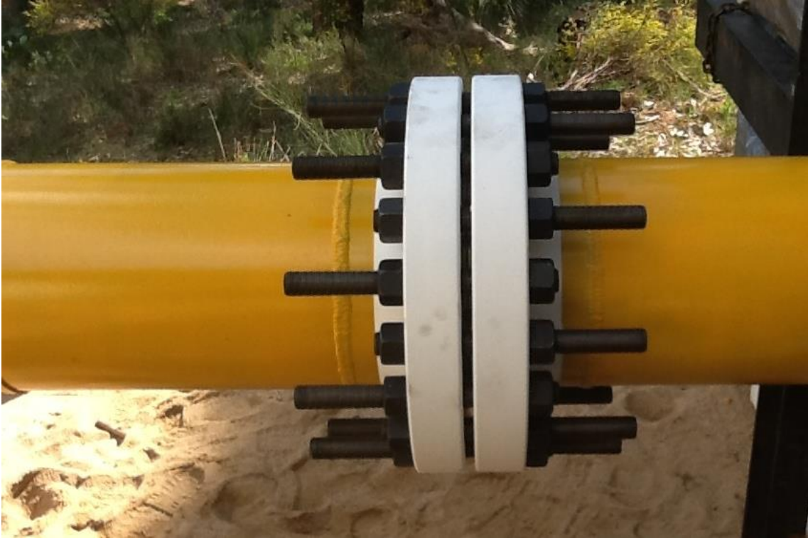
Figure 3.3: Flange connecting spools with a standardized amount of bolts (OSTS)
