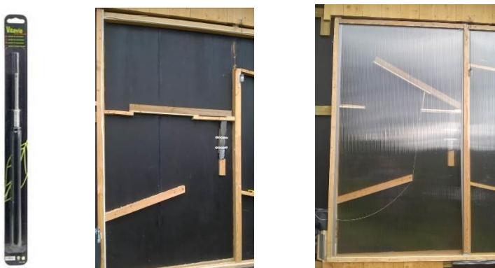
Figure 8. The thermal expander (Hageweb, 2015) and the closing mechanism.
