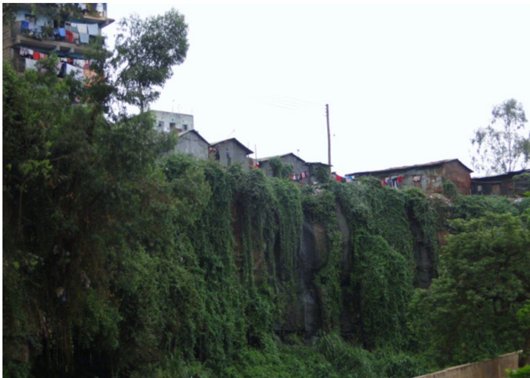
Photo 4.1: Housing structures built on edge of quarry (MST, 2013)
