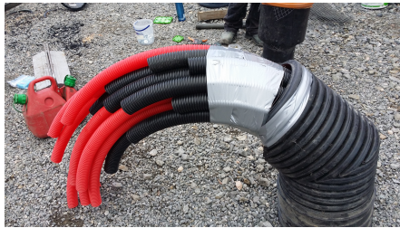
(e) A 300mm 90 degree bend with 50-60mm pipes inserted.
