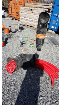
(c) Nozzle construction site.
