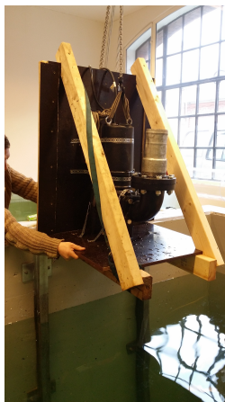
(b) Installing the pump
