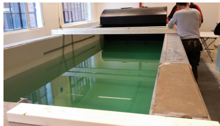
(a) Constructing the work platform
