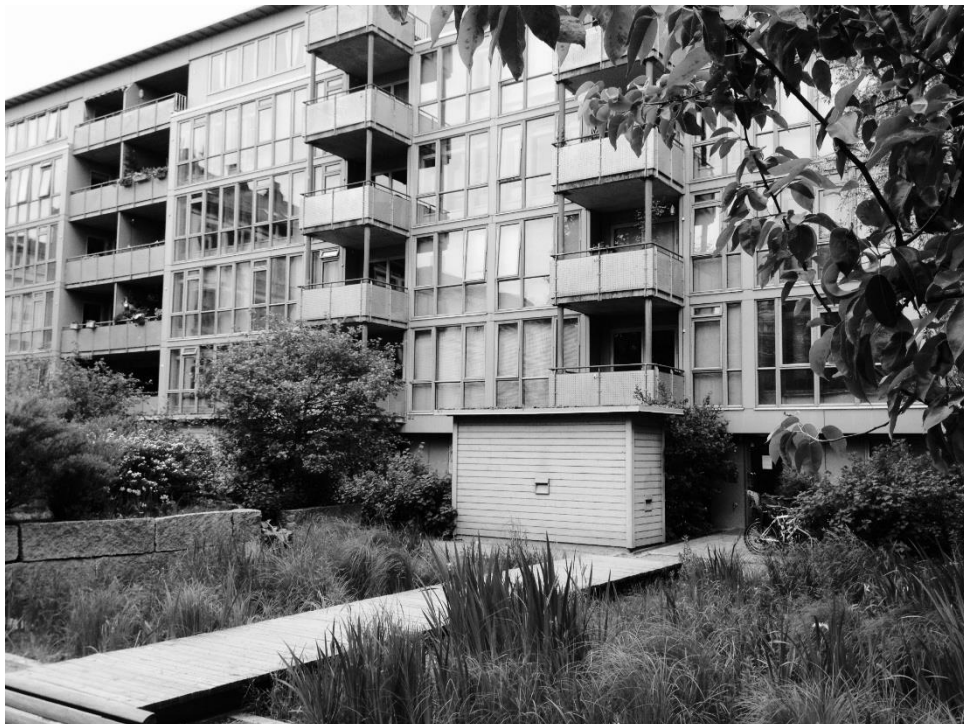
Figure 11, Picture taken in 2014 of the constructed wetland in front of the KL building. The elevated area to the left is the top of the biodomes.
