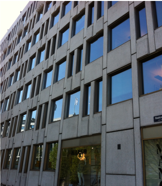
Figur 31: Haakon VII's gate 10, bevaringsverdig fasade (bilde fra befaring, april 2014).
