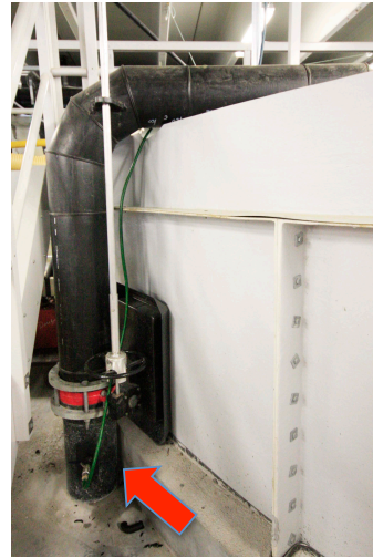
FIGURE 23: THE RED ARROW MARKS THE VALVE, FROM WHICH SAMPLES FROM THE FISH TANK INLET PIPE WERE TAKEN.
