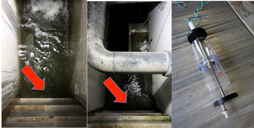
FIGURE 22: (LEFT) RED ARROW MARKS THE SAMPLE SPOT WHERE SAMPLES WERE TAKEN FROM THE EFFLUENT OF ONE OF THE TWO DEGASER; (MIDDLE) RED ARROW MARKS THE SAMPLE SPOT OF THE SECOND DEGASER; (RIGHT) WATER SAMPLER USED TO TAKE SAMPLES OUT OF THE WATER COLUMN FROM INFLUING WATER OF THE DEGASER INTO THE PUMP SUMP.
